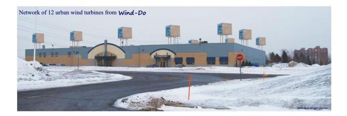
A company having a building of 80 meters by 40 installed on its roof 12 urban wind turbines each one harnessing 30 square meters of wind. The owners chooses urban wind turbines because his building is within 100 meters of a residential district. They also chooses a distribution of medium size wind turbines as their consulting engineers estimated that this way no modification would be necessary to the building structure.
